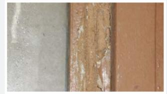
Damaged or eaten wood, or wood with mud tubes, which indicates the presence of termites.
